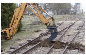
Railway Cribbing Buckets are a necessity for almost any contractor or railroad working in track maintenance.
