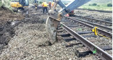
DymaxRail Cribbing Buckets for excavator machines are 8 inches wide but feature a longer tip radius and are built to last.
